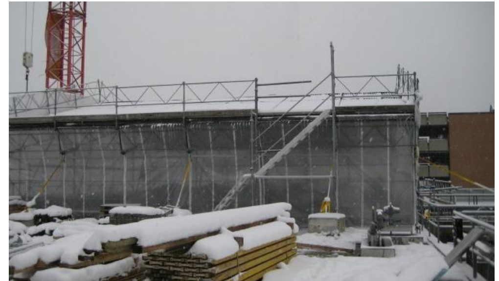
ozone contactor under construction
